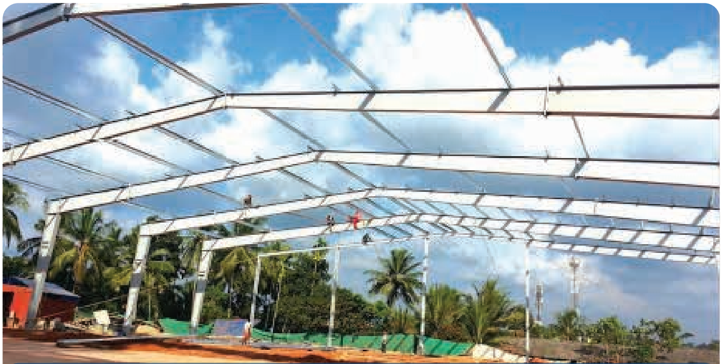
Warehouse, Near Ramanattukara.
