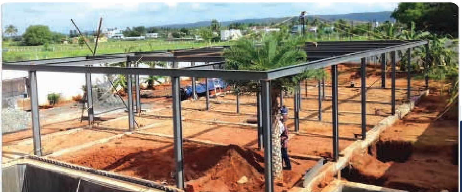
Paramount Textile Mills, Madurai Paramount Textile Mills, Madurai
